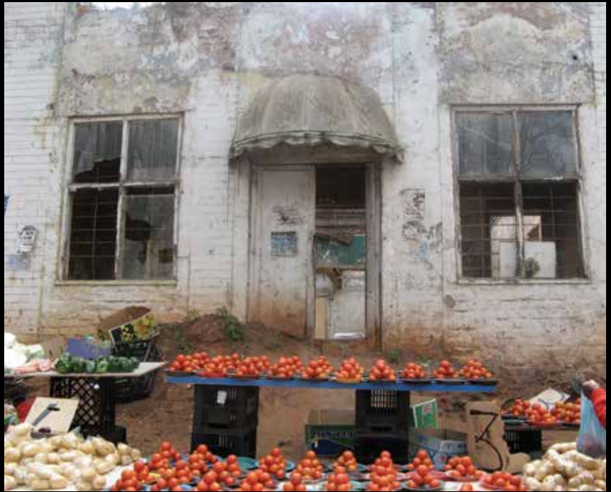
A dirty building where people sell their produce along Abel Street in order to earn a living. This image reflects the lack of adequate selling spaces for vendors in Hillbrow.
